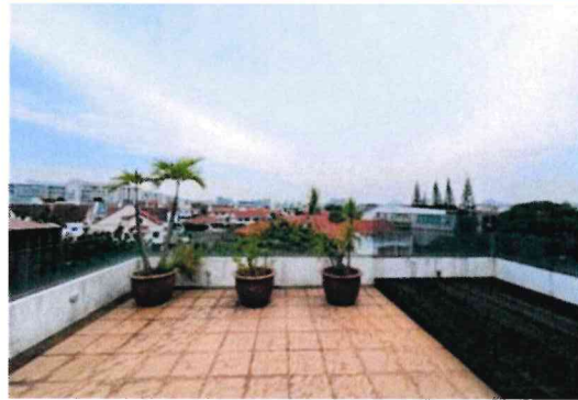
Open Roof Terrace
