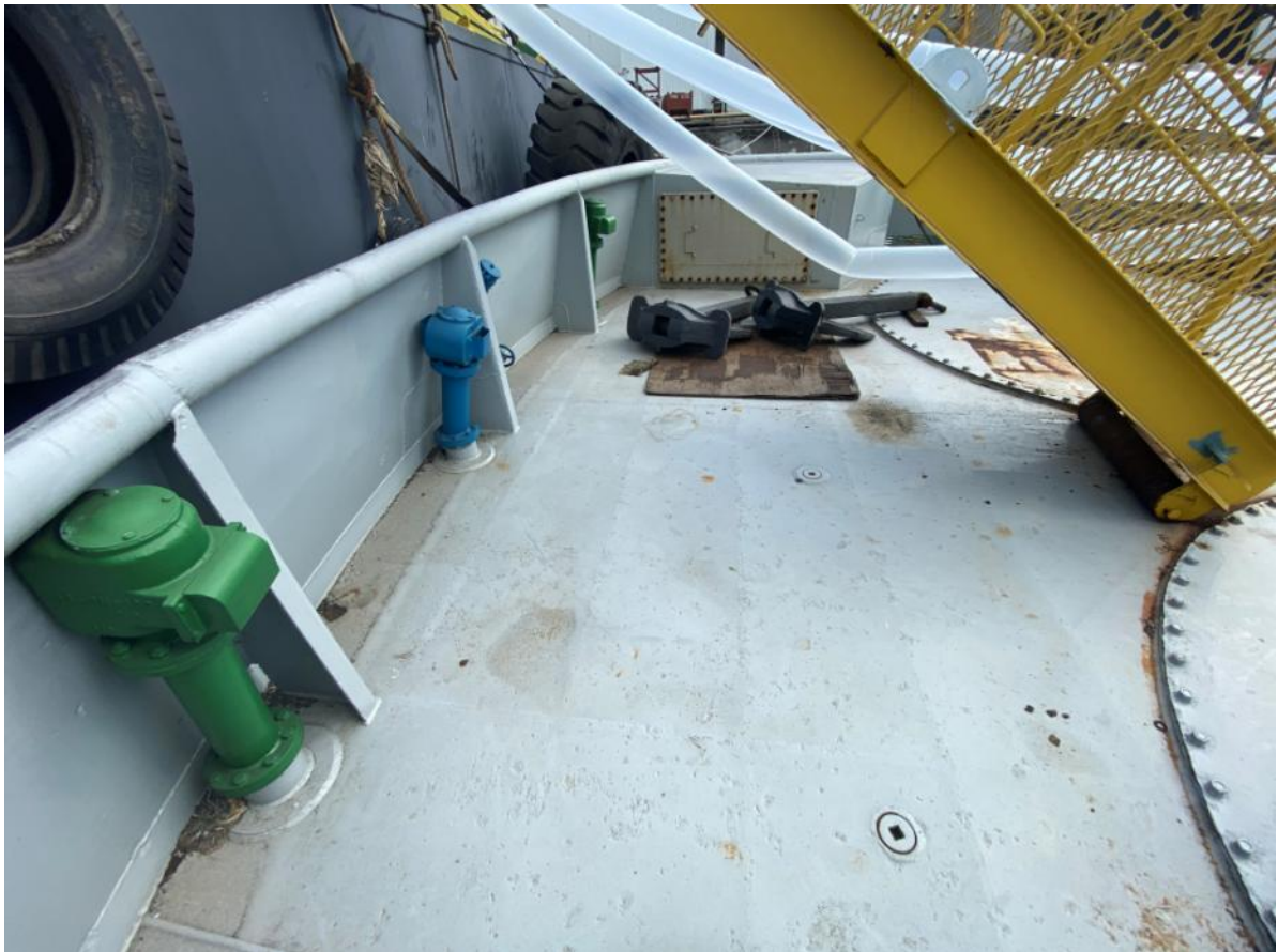
022. Good deck plating condition.
