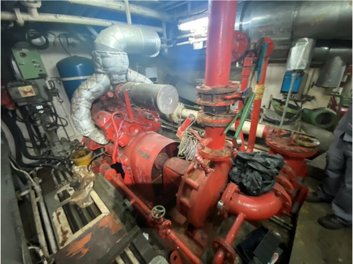
093. Engine driven FIF1 pump.
