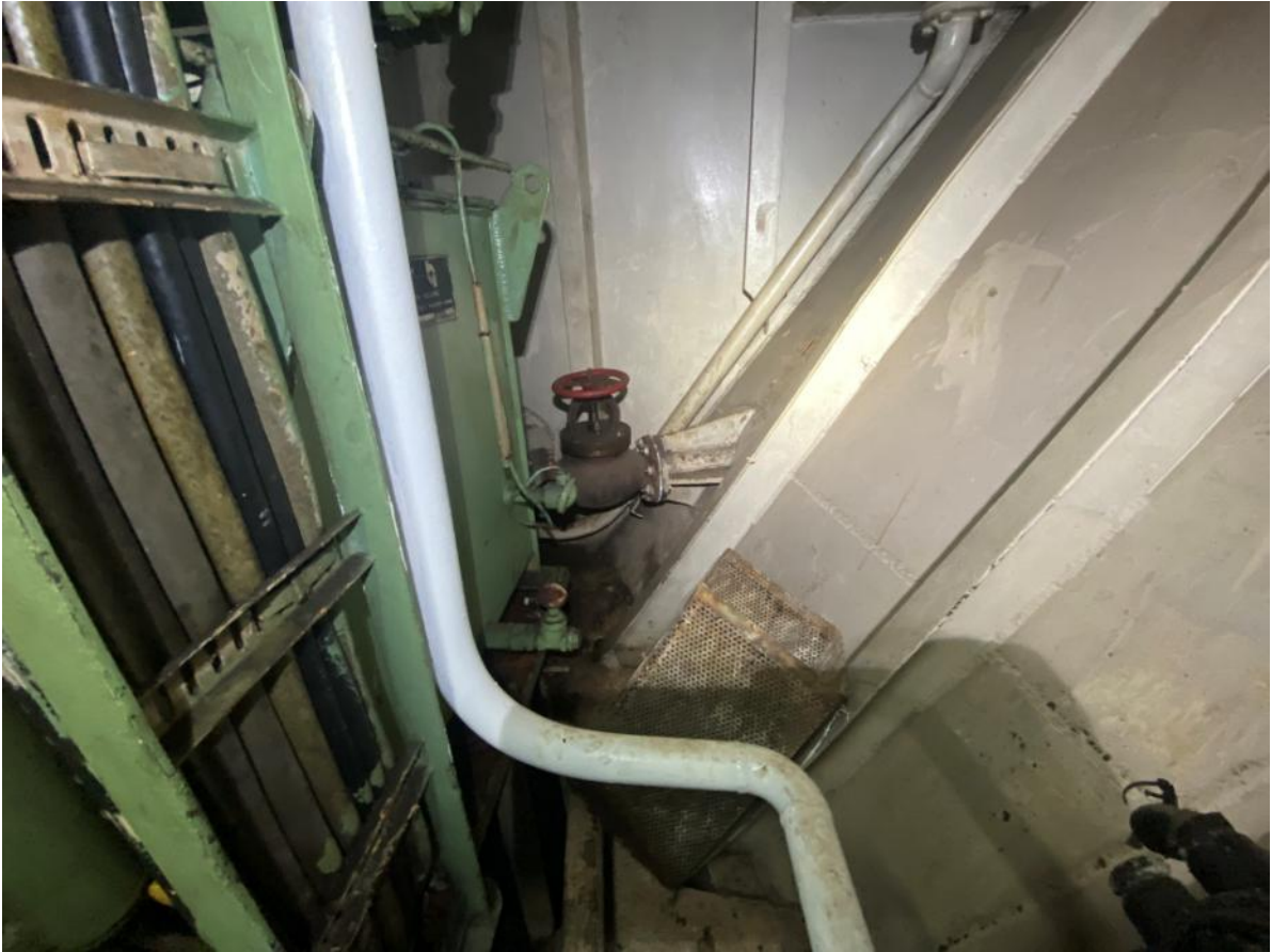
079. Overboard valves appeared newly replaced.
