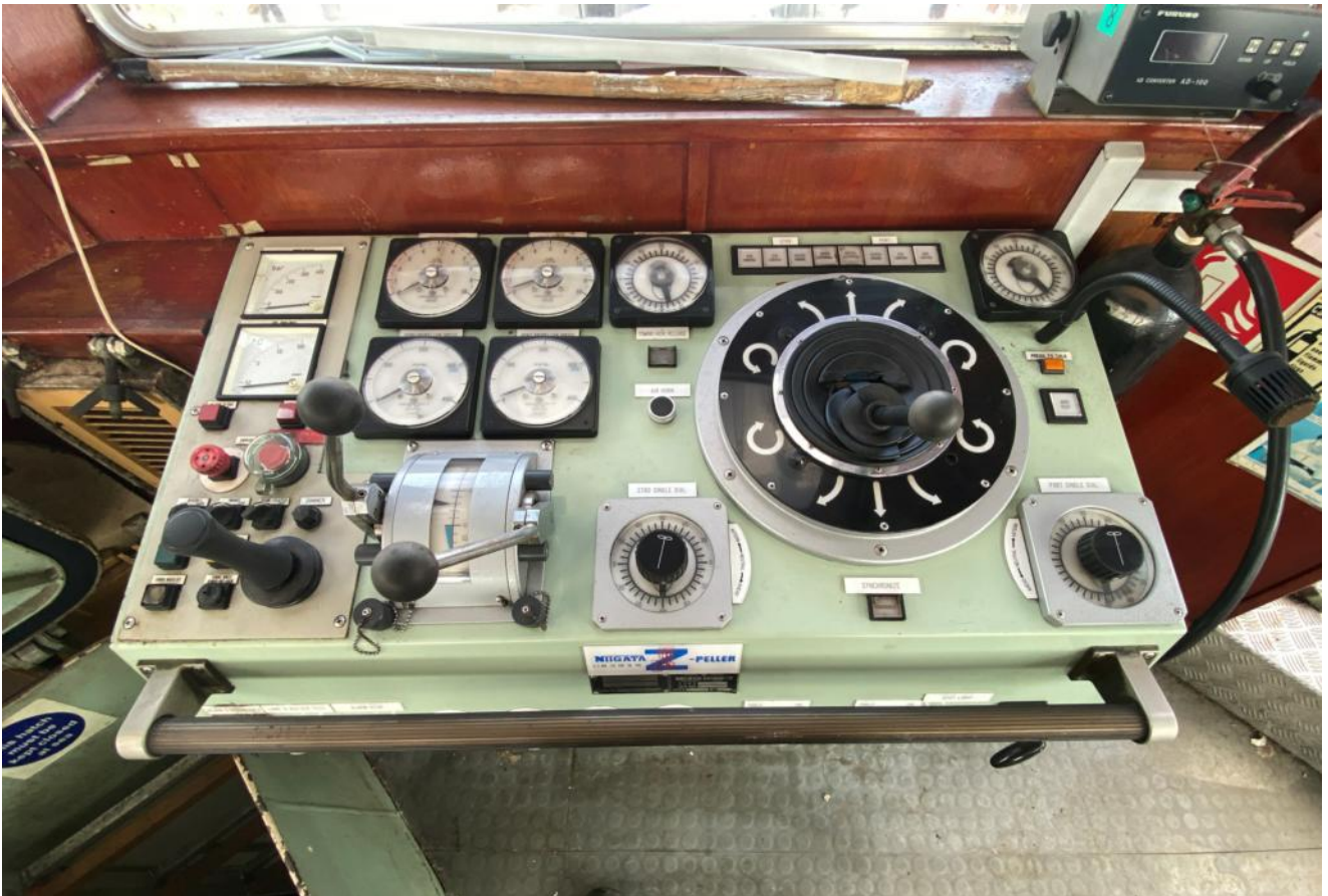
055. Aft facing steering and winch control console.
