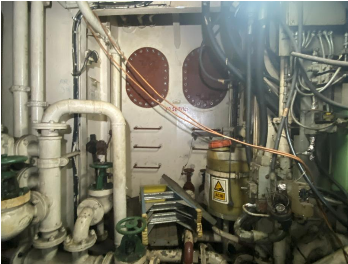
081. Fuel service tanks.
