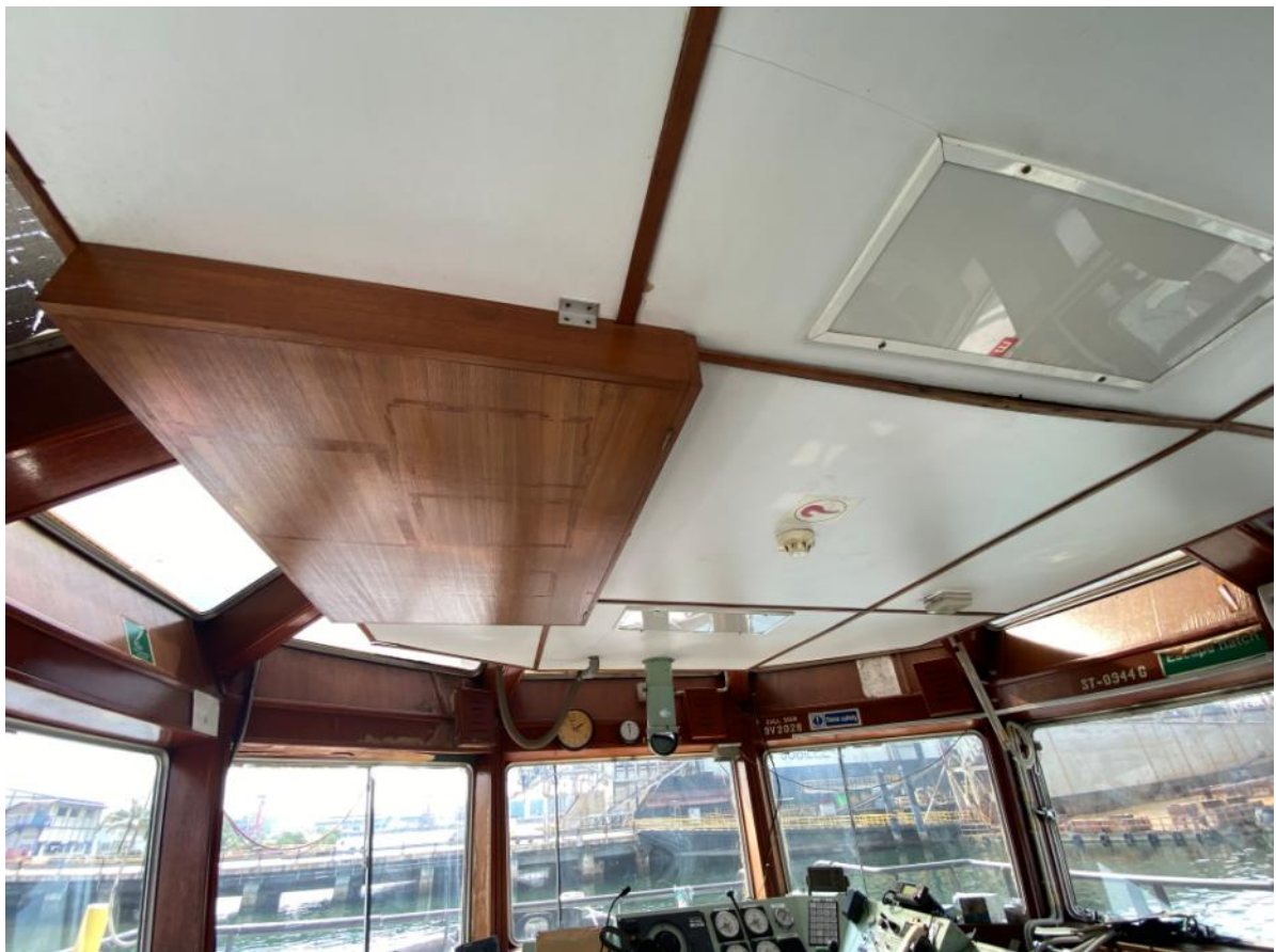
036. Wheelhouse ceiling panels in good condition.
