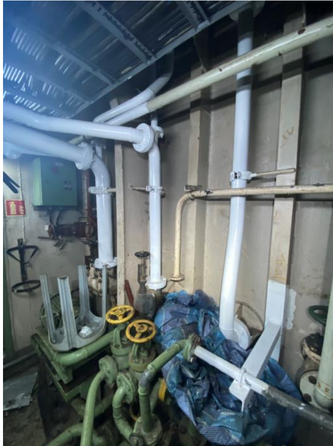
089. Some replaced piping.
