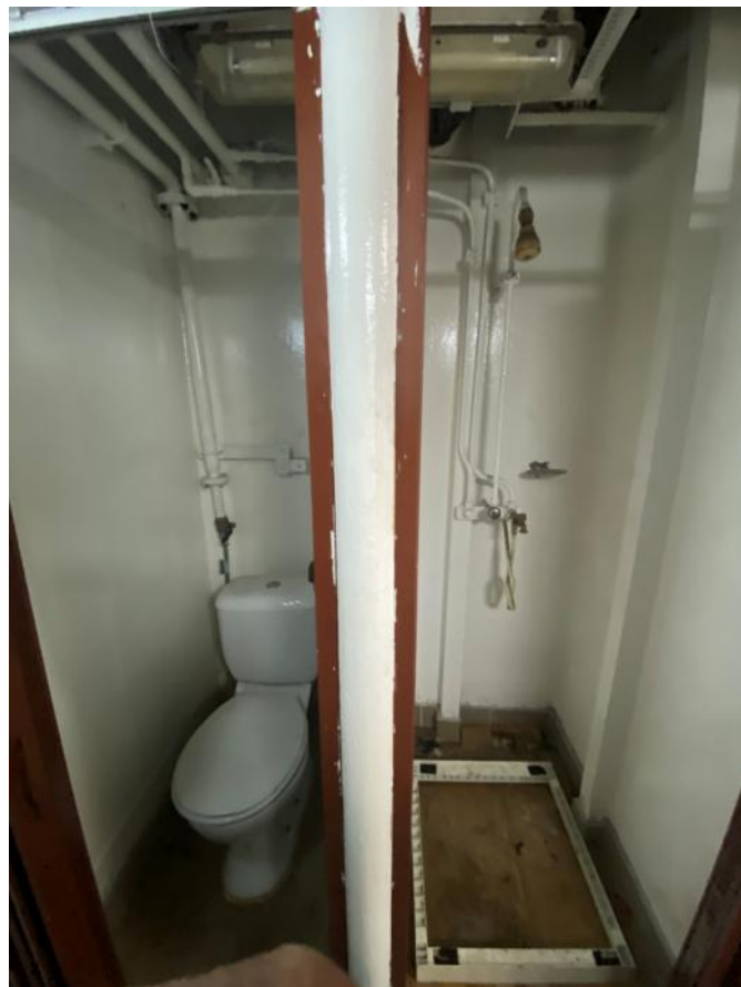
070. Separate toilet and shower cubicles.
