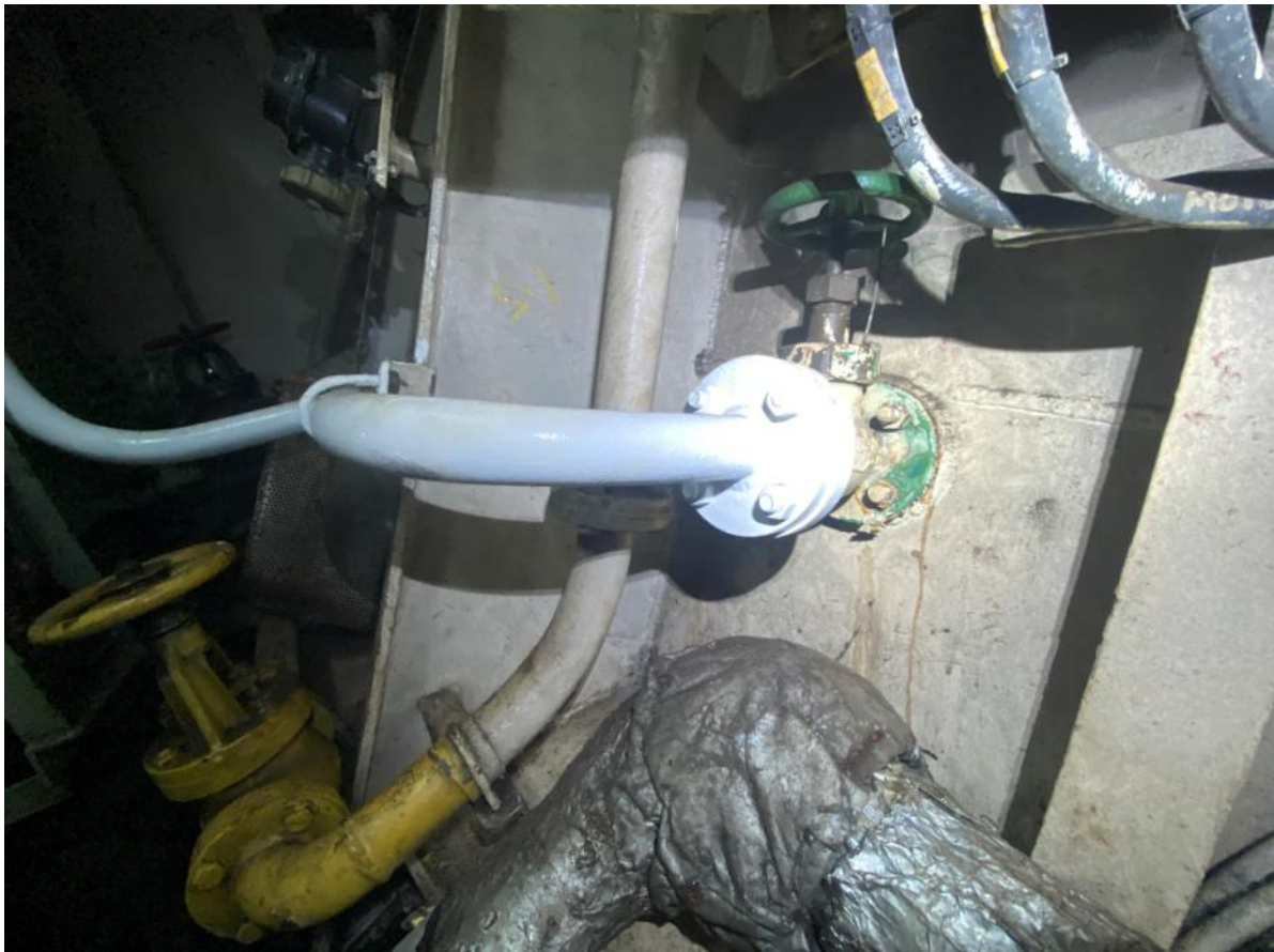
078. Replaced sw overboard piping.
